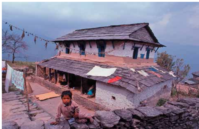
Left Nepal: the main material used for the houses in the Nepalese mountain village Dham-pus, is slate. It is used in partially white-washed walls and for the roofs. Windows, supports and roof brackets are made of carved wood.
